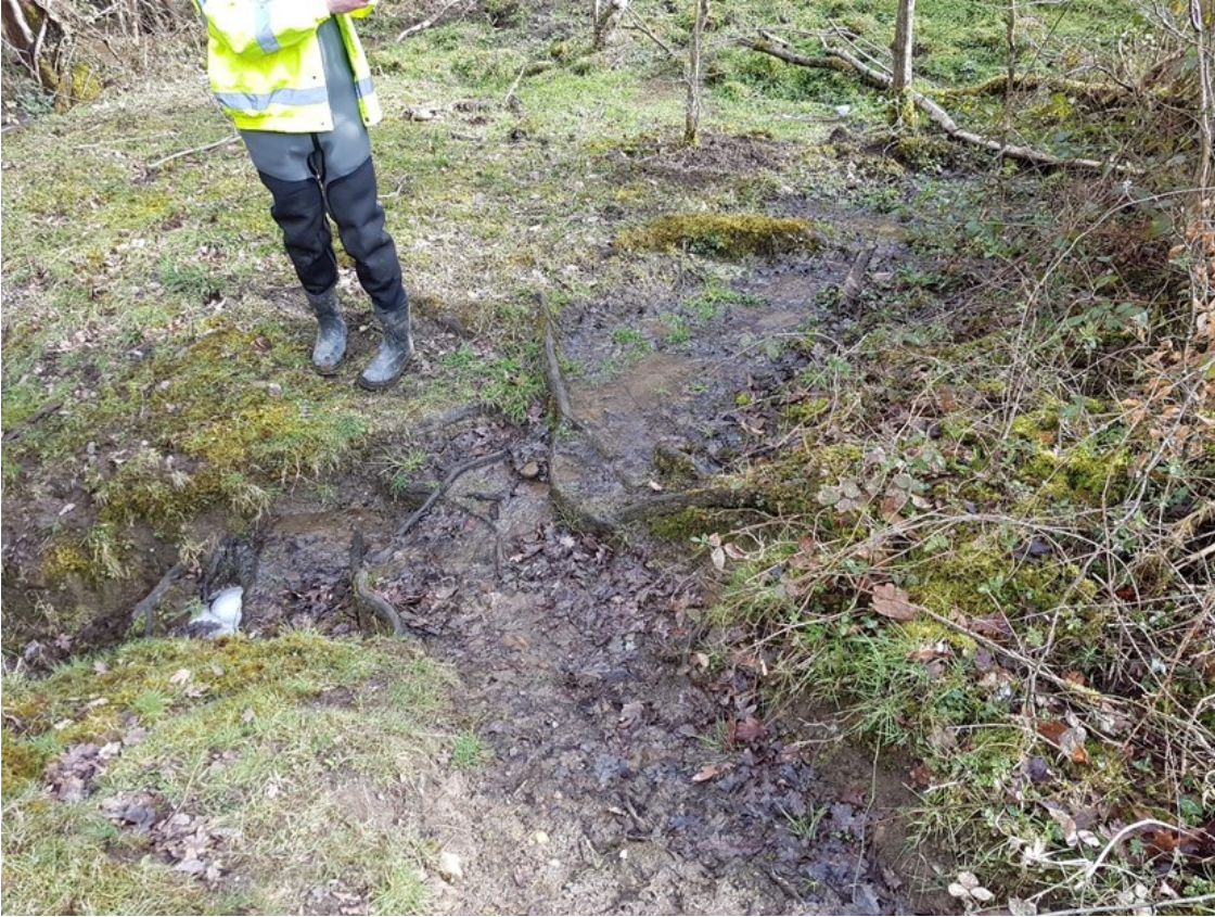
Saturated made ground/seepage
