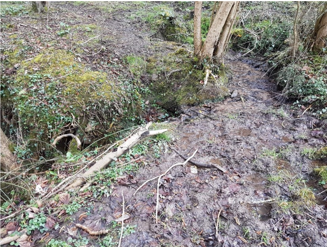
Saturated made ground/seepage
